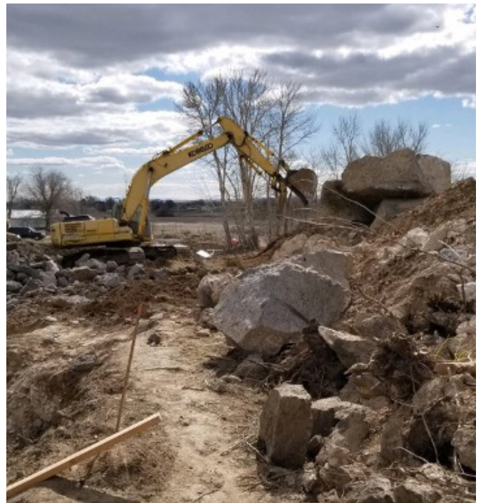
Tailrace powerhouse grubbing & clearing at the MC6 hydroelectric construction site
