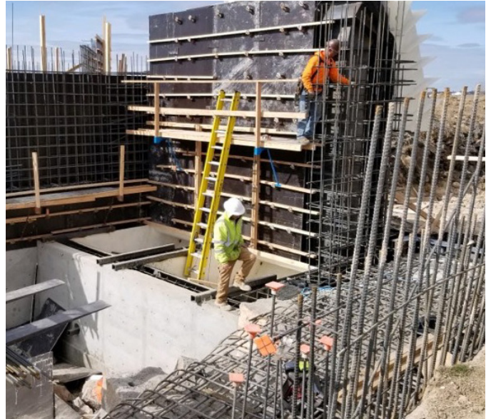
Construction workers on the MC6 hydroelectric project install the bypass intake concrete and siphon
