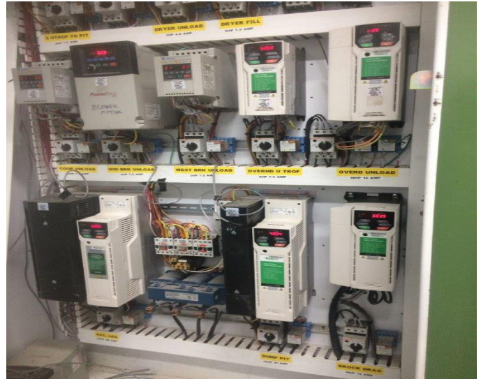
Variable Frequency Drive (VFD) system improves energy efficiency in Smiley farm operations
