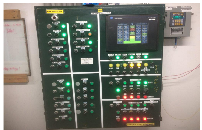
Control panel for Smiley Farms' VFD system
