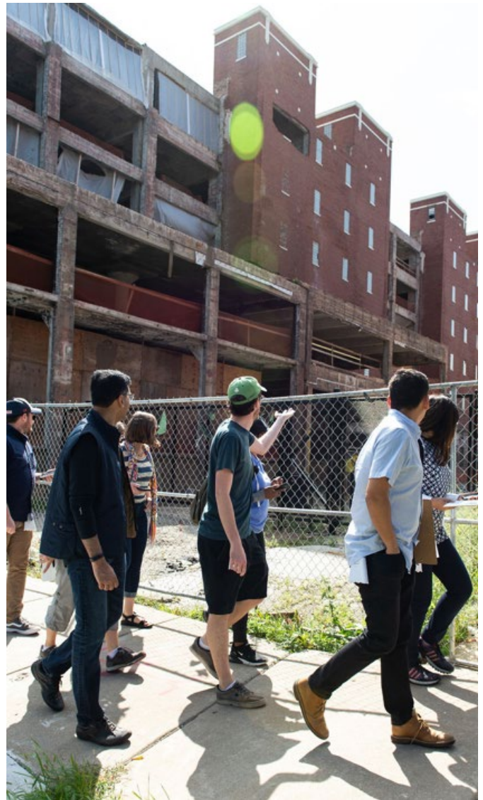
Figure 12: Volunteers and community partners with Neighbors for Environmental Justice at a community air quality monitoring day in the McKinley Park neighborhood, 2019
