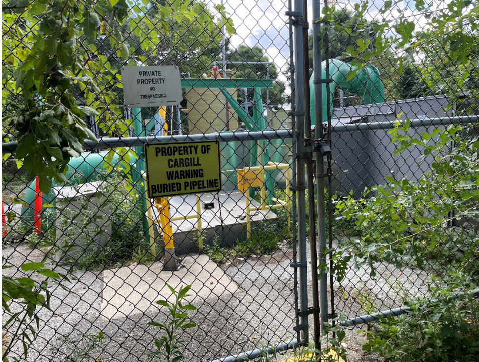
FIGURE A.6. View of Cargill Lake Michigan Intake Pump House. Photo by Carolyn Marsh, BP & Whiting Watch.
